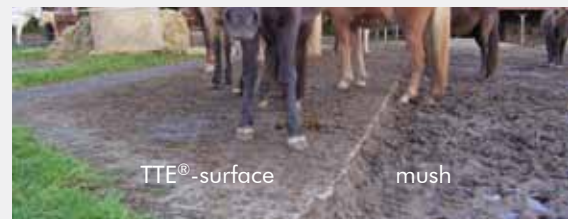
This bad weather surface was built directly on mush. Partial paving may be extended any time.
