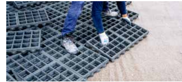
Laying of the TTE® elements on the fine matrix (installation aid).
